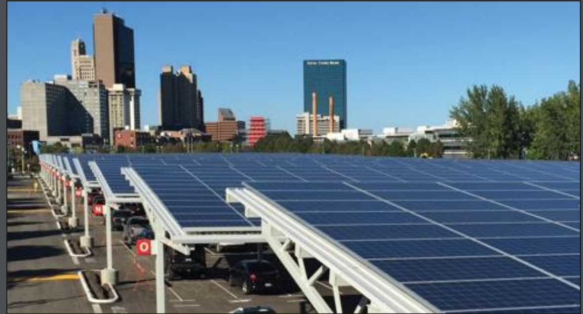
Owens Corning Interior renovations/ solar field
