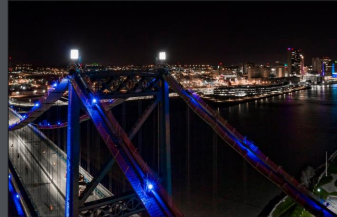
Anthony Wayne Bridge
