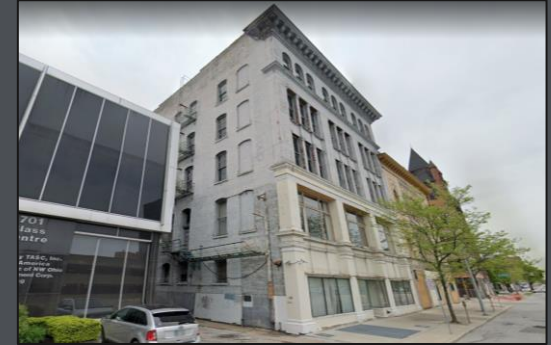
Lofts on Jefferson
